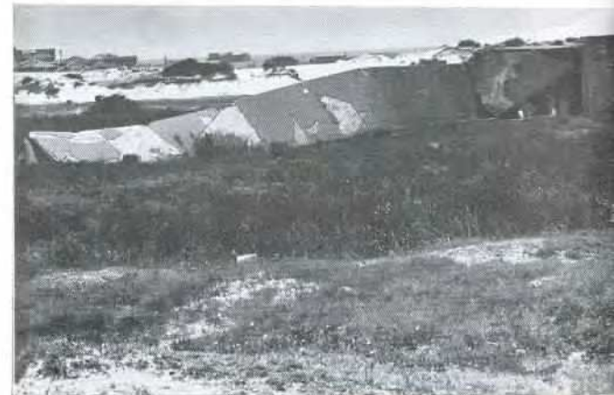
Just before the site was finally covered with brick houses, this wall was the one remaining sign of Maroubra Speedway.
